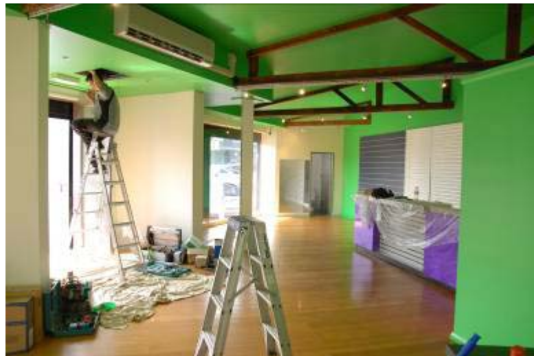
The new location was repainted to DCW specifications
